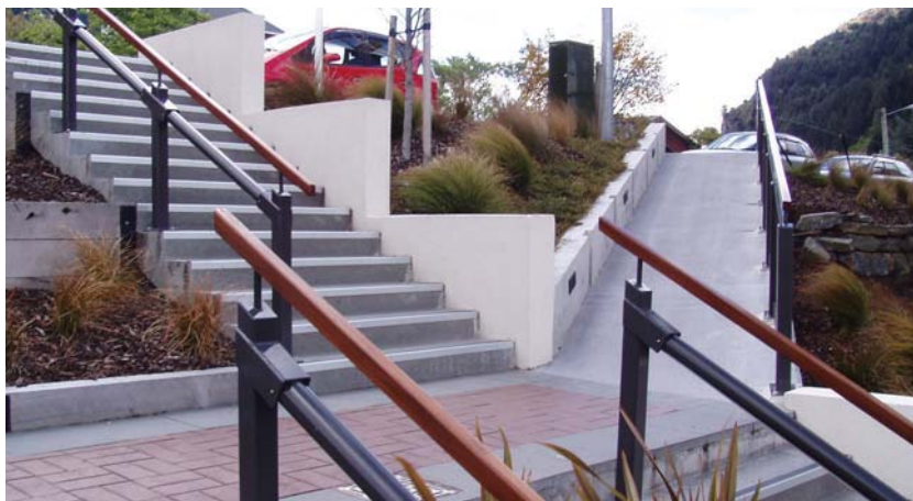
Photo 14.17 – Choice of ramps or steps, Queenstown (Photo: Tim Hughes)
